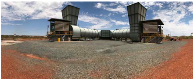
Figure 2. Full turnkey installation project for a gold mine in Tanami (Australia).
